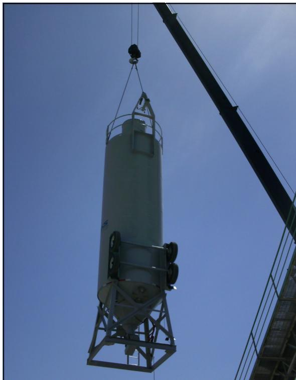
The crane operator will pull up the silo. The legs and base of the silo are strong enough to support the silo being lifted. Once the silo is vertical the crane will set it down in the desired location.
